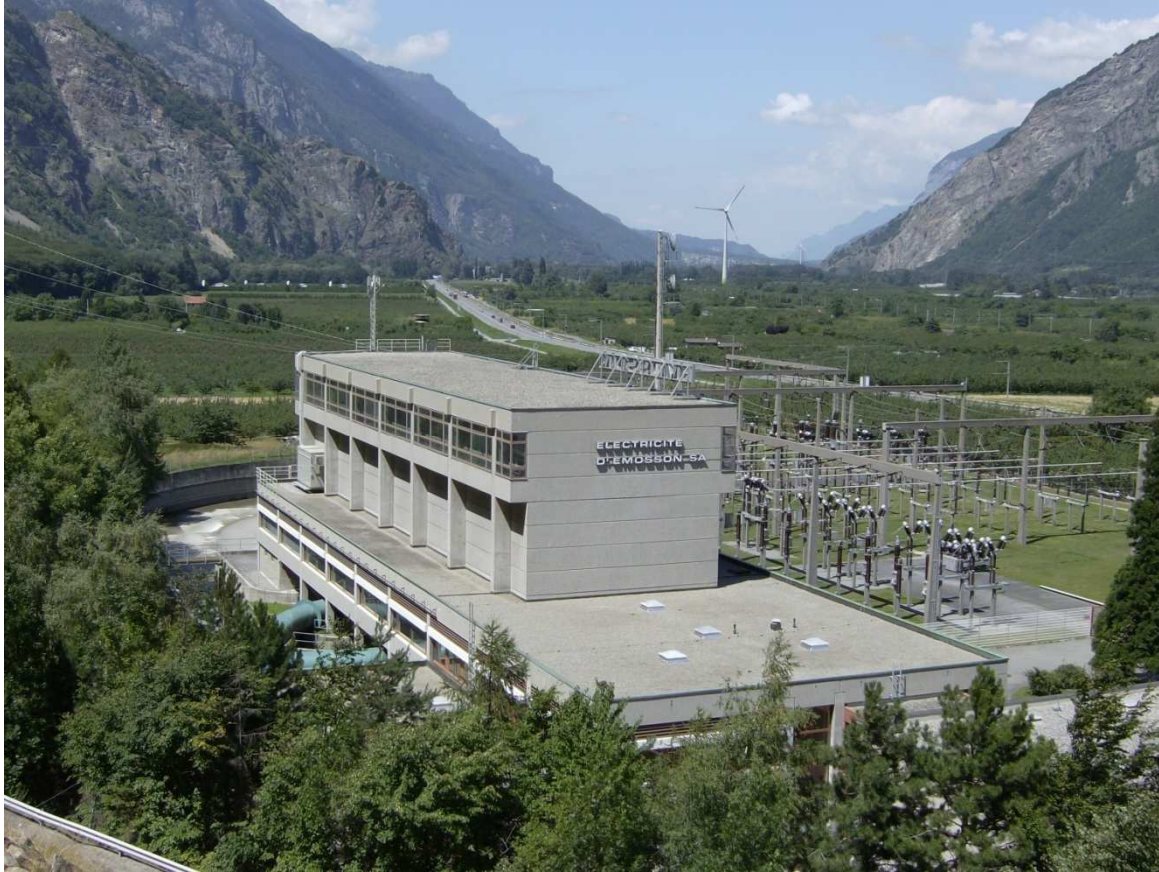
Figure 4 Power house of 170 MW La Bâtiaz HPP.
