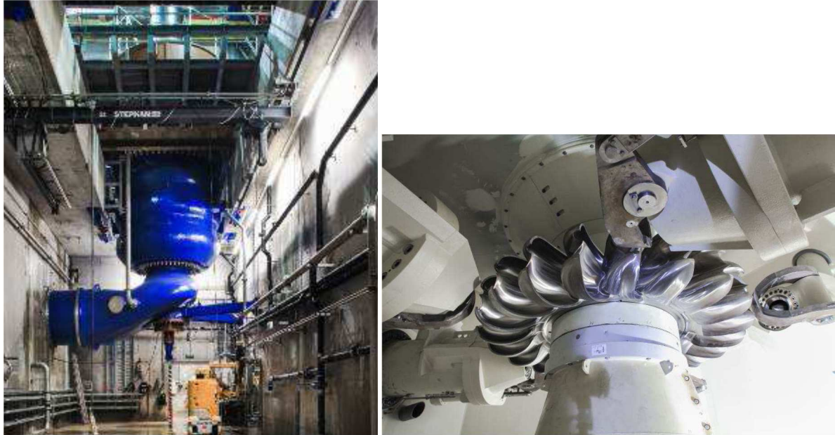
Figure 6. Pictures of the new unit 5 of Veytaux II including 5 stages storage pump (left) and Pelton turbine with 5 injectors (right), [8].
