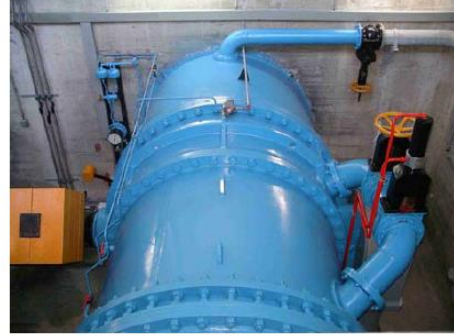
Figure 2. Penstock protection valve of DN1800.
