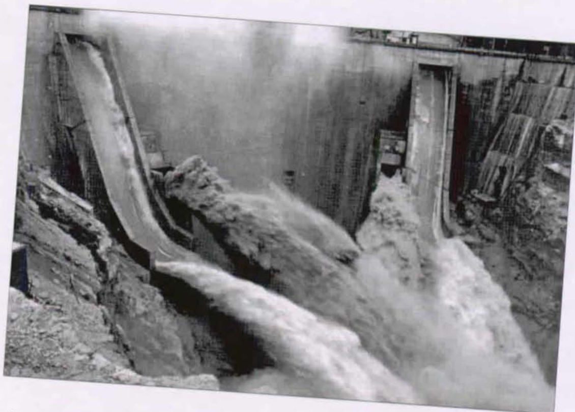
Photo 1 A 5'000 m 3 /s flood discharge at Jiroft dam (Iran): combination of highly sediment-laden flow, issuing from intermediate outlet works, with clear water coming from the ski-jump overflow structure (Photo B. Hagin, Stucky Ing. Conseils).
