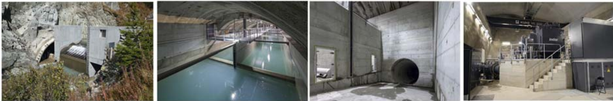
Figure 1 Picture of the intake, the silting chamber, the forebay tank with the inlet of the headrace tunnel and the machinery cavern of KWGO SHP, source: FMV
